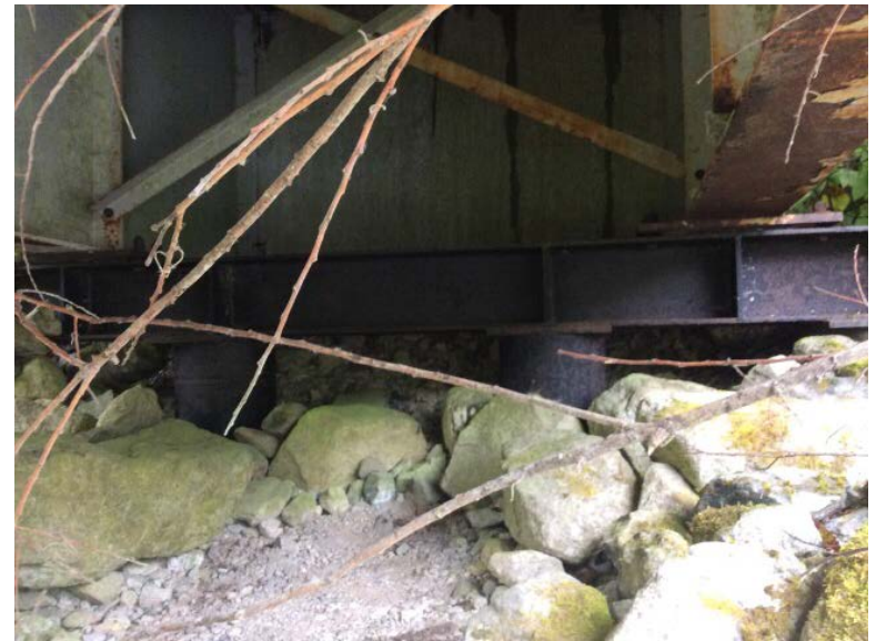
Right Bank Abutment when facing downstream
