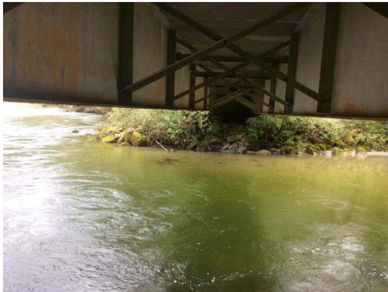
Right Bank Abutment when facing downstream
